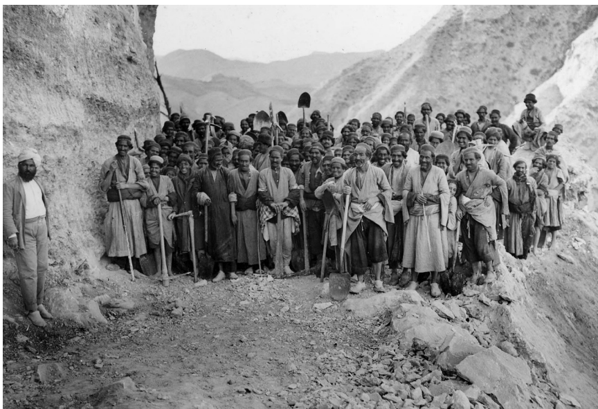
Figure 2. Construction of the Gach-qaraguli (Gachsaran) Road, 1909
